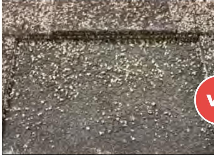
**Standard Asphalt Roof With Severe Granule Loss**
